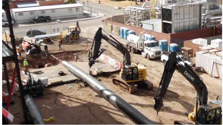
Figure 7 – Pull in of Pre-insulated PE-RT Pipe in Horizontal Bore
