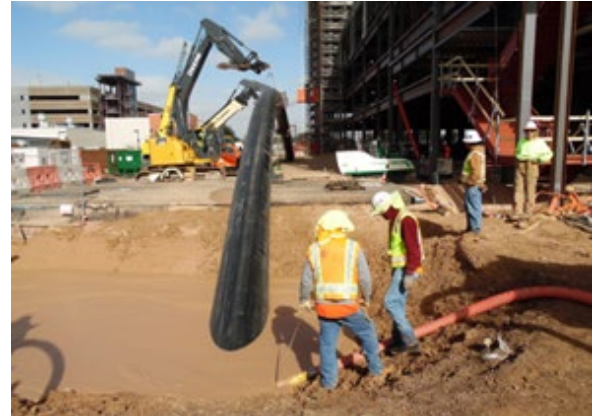
Figure 1 – Pre-insulated PE-RT pipe. Banner Medical Center, Tucson AZ
