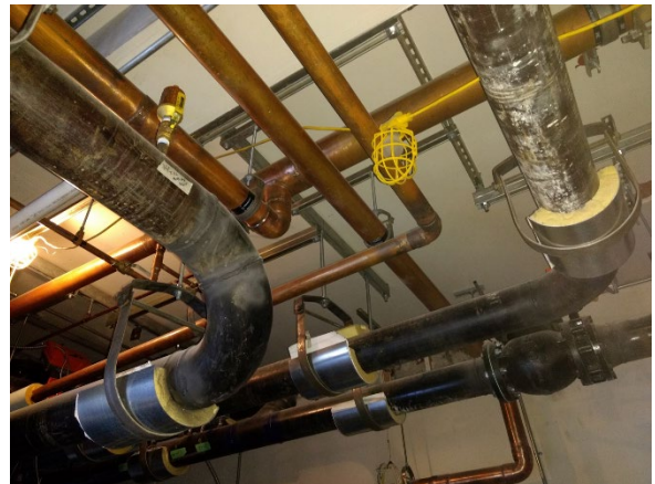
Traditional Commercial Building Pressure System Piping Systems largely include Copper, Steel, and Ductile Iron Piping
