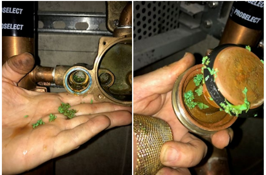
Residual plastic slivers and chips will clog fittings/devices if not properly removed
