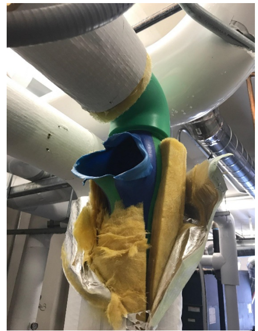
Example of a PP-R Pipe Failure due to prolonged overtemperature
