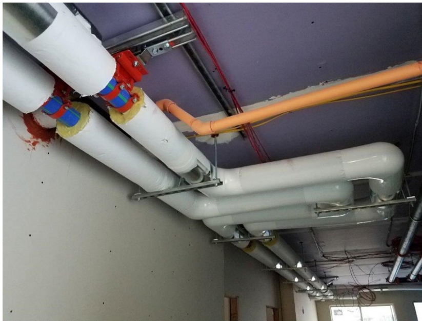
Example of Installed 'U' Bend Thermal Expansion Compensation Assembly
